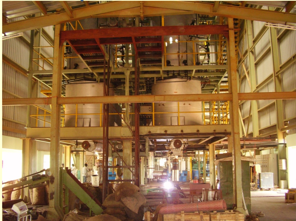
BMC GASIFIER PLANT(1700Kgph)
